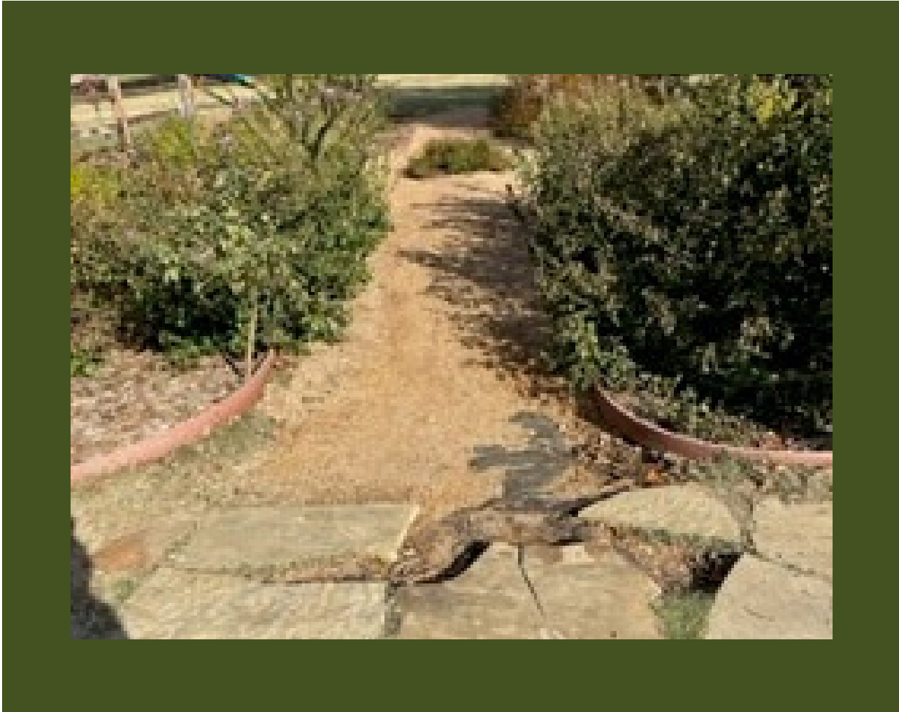
CRUSHED GRANITE REPAIR AT HARRY MYERS PARK
